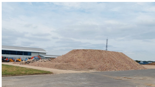
Groundworks by Blanchard Wells on the Industrial Area between the Coastguard Hangar and Daedalus Drive
